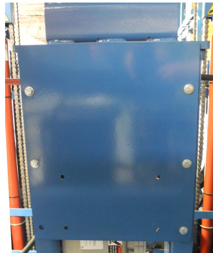
Cover/Stiffener Plate installed properly
